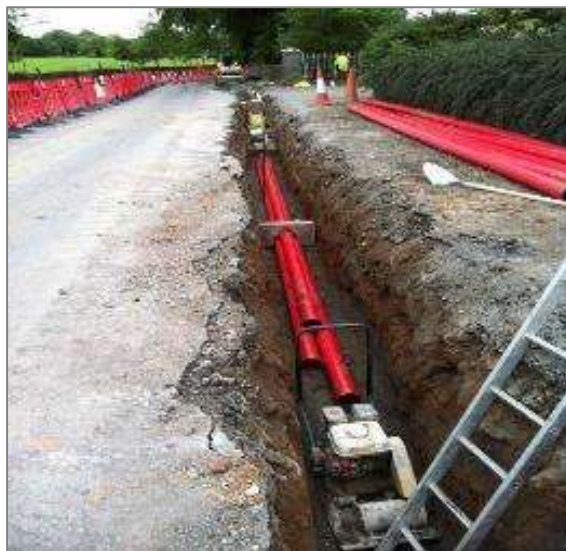
Figure 2 - Typical 110kV Underground Duct Installation
